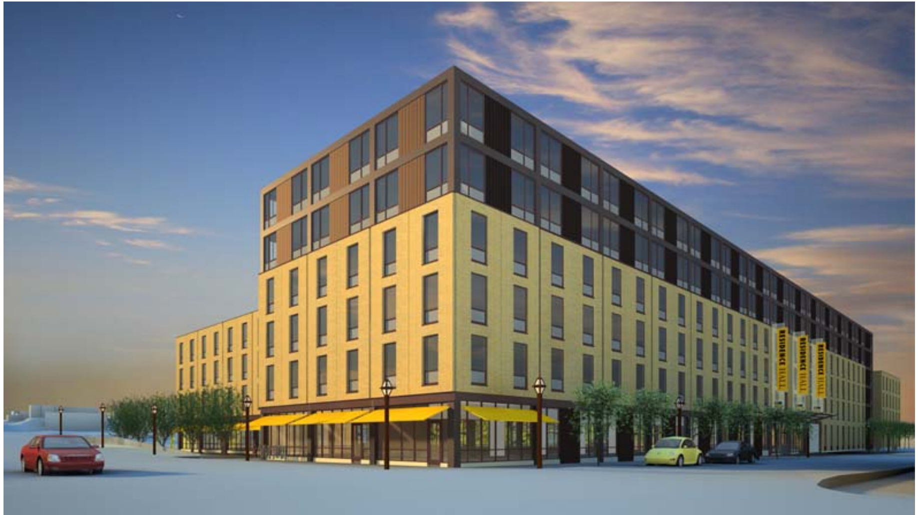
View Looking NW from Intersection North Avenue and Cambridge Avenue
